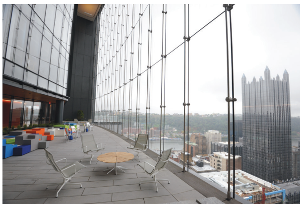
The 33-story tower has a double-skin facade and operable "poppers." A terrace and "indoor park" with radiant-heated floors occupy the building's 28th floor (above).
